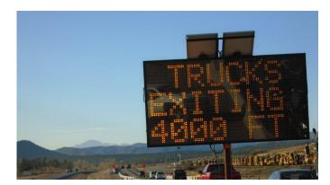
farther back in the corridor is triggered and will light up a sign to warn motorists in time to slow down and yield to the truck.
